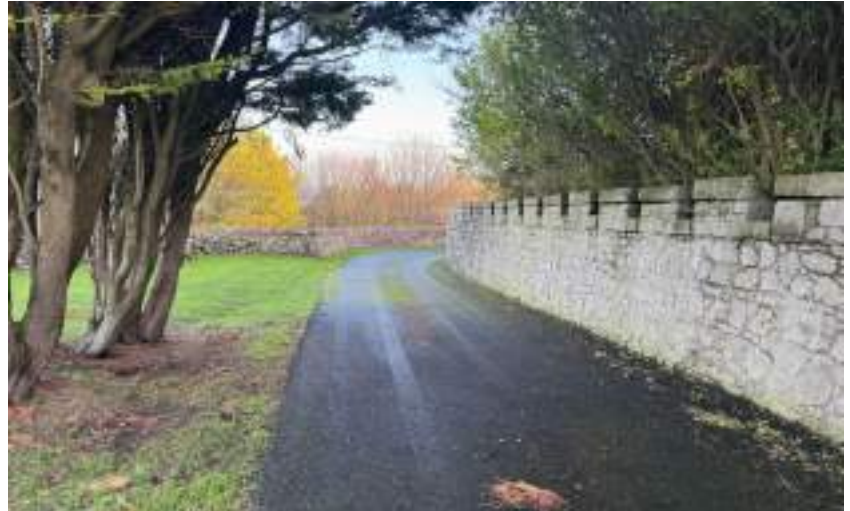
Photographic Plate 1 – Site access road from Lizard Lane looking east. Marsden Hall boundary wall to rhs of picture.
